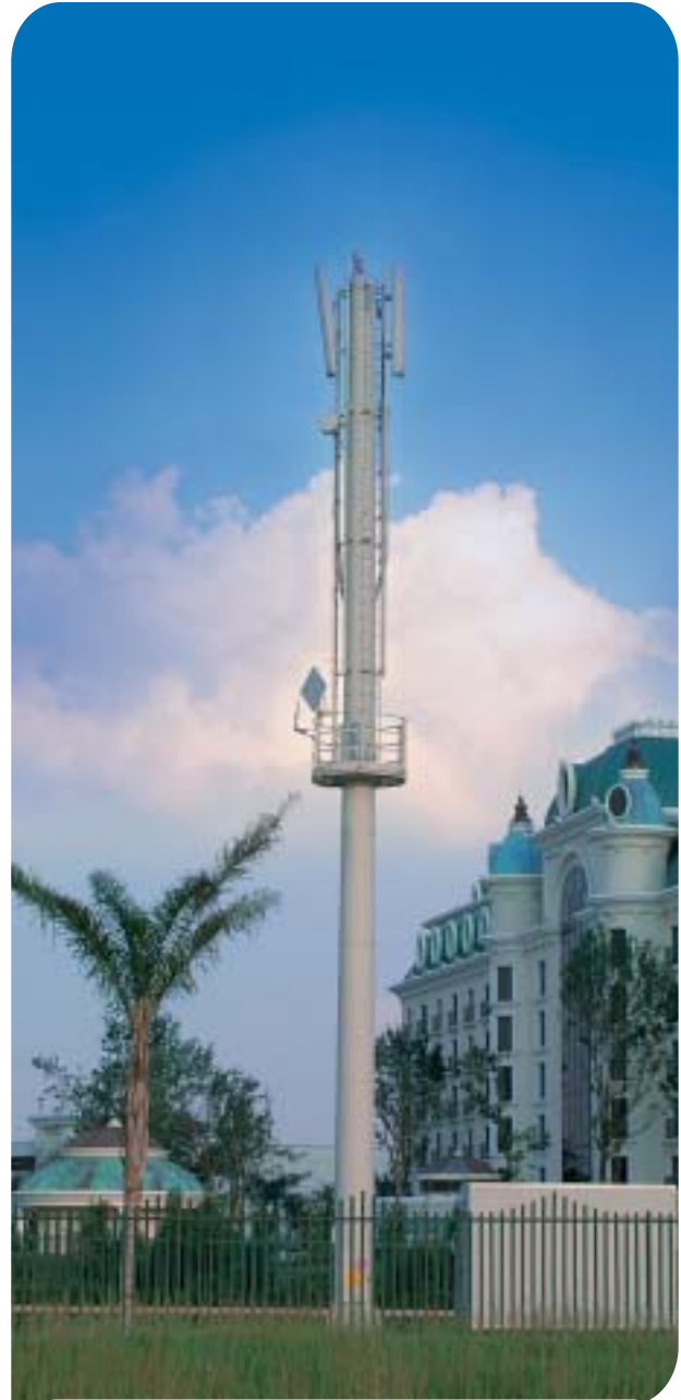
Vodacom base station at Caesar's Palace, Gauteng
